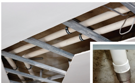
Shallow flue voids & flue kit
