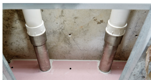
Shallow flue voids & flue kit
